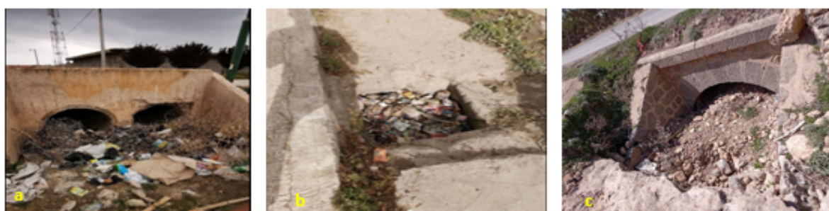
Figure 8. Malfunctioning of the urban drainage system observed in the field: (a) Heavily loaded discharge canal, impairing proper flow. (b) Sewer blocked by solid waste, observed in a residential neighborhood. (c) Drainage structure clogged with poorly sorted coarse sediment deposits (silt, gravel), hindering flow and promoting overflow.
