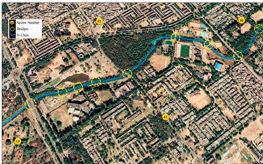
Figure 3. Bridges (encircled yellow) allowing the vehicular and pedestrian traffic flow without disturbing the streamflow in N-choe Source: Developed by authors from the Google Earth imagery
