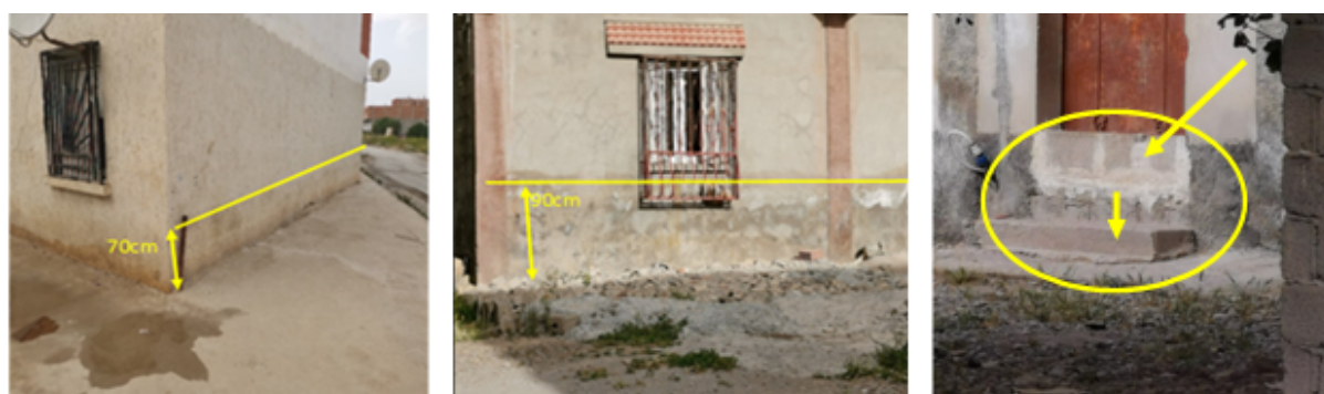
Figure 11. Effects of the June 2023 flood on buildings and residents' individual adaptations: (a, b) Flood marks visible on the walls of a dwelling (June 2023). (c) Raised doorway threshold installed to limit water intrusion.
