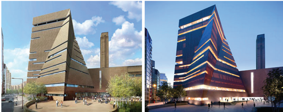
Figure 2: Proposal design for expansion of Tate Modern museum to officially open in 2016 - Herzog & de Meuron, London, UK
