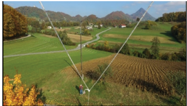
Figure 13. Transporting leader cable for electrical grid
