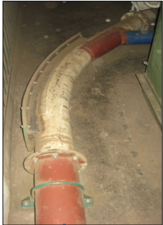
Figure 1: Knee reinforced with PE 1000
