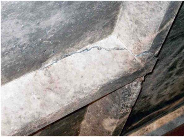
Figure 3: Inclined crack in the reinforced-concrete rib (left) and peeling of concrete on the top support ring caused by fire (right)
