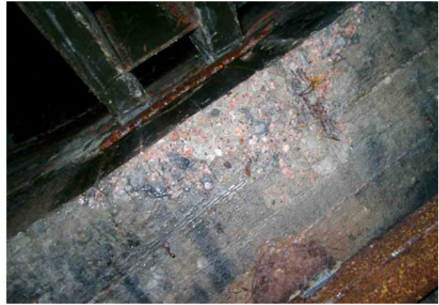
Figure 3: Inclined crack in the reinforced-concrete rib (left) and peeling of concrete on the top support ring caused by fire (right)
