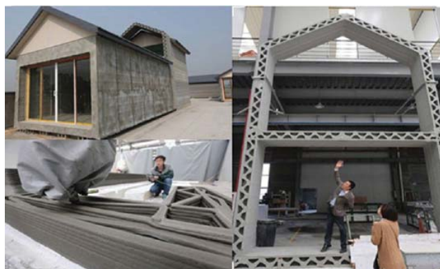
Figure 1: WinSun building and wall construction (China, 2014) [6]
