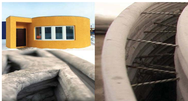
Figure 2: Demonstration building in Stupino and the construction of its walls (Russia, 2017) [8, 9]
