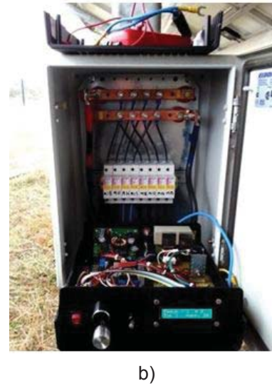
Figure 7: Starting «Intelligent device for selecting maximum power and matching photovoltaic arrays» (a – structural connection scheme, b – installation in the circuit breaker panel of a solar power station) 1 – evenly lit array, 2 – partially shaded array, 3 – intelligent device for selecting peak power and PV matching, 4 – MPPT controller
