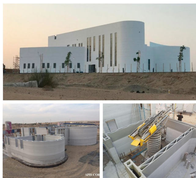
Figure 1: Two-story building erected by APISCOR in Dubai in 2019 [10], [11]
