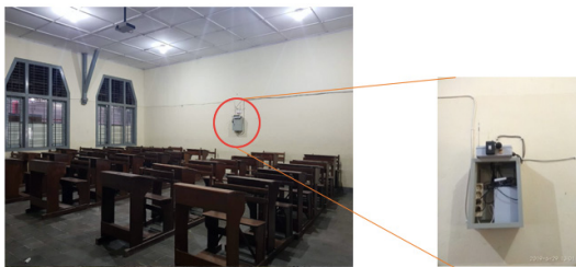
Figure 17: The installed sensor in the selected position in the R40 classroom
