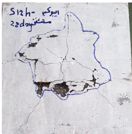
Figure 16: Failure pattern of HH-56
