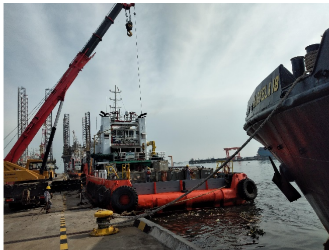
Figure 2. Lifting activity mobile crane with supply boat at Marunda Jetty
