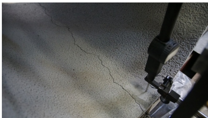
Figure 8. Crack of the width of 2mm inside the specimen #2
