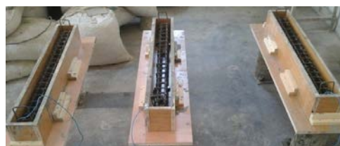
(b) Steel reinforcement cage inside the wooden mold
