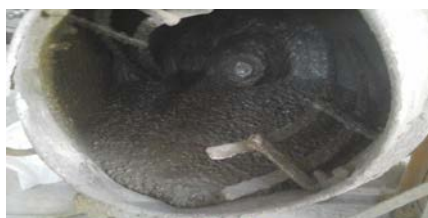
(c) Mixing of concrete
