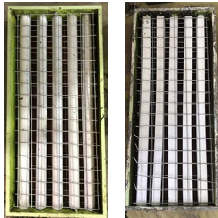
Fig. 5. Slab preparation before casting
