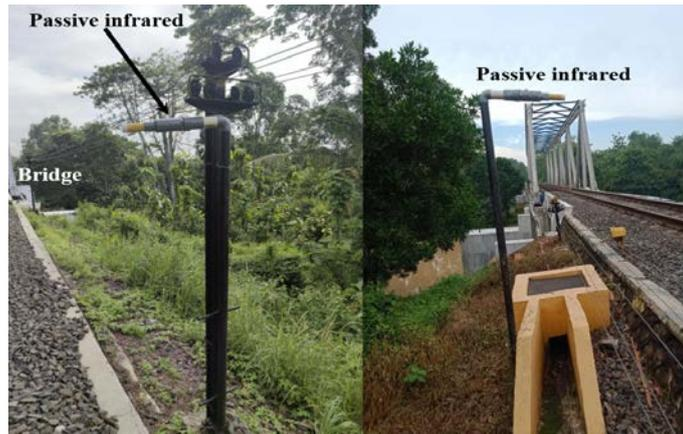
Fig. 4. Location of passive infrared sensors relative to the steel structure railway bridge
