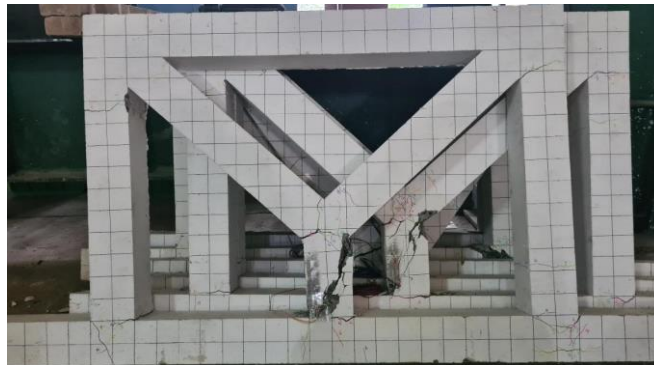
Fig. 17. Failure of EBF shear link of 25 cm structure
