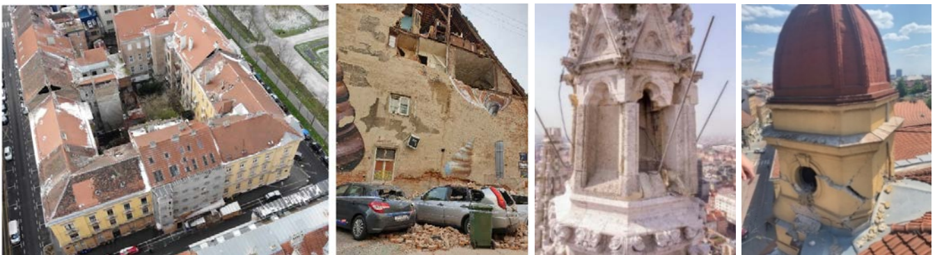
Fig. 2. Zagreb earthquake (source: HCPI, 2020; AIR-RMLD d.o.o.)
