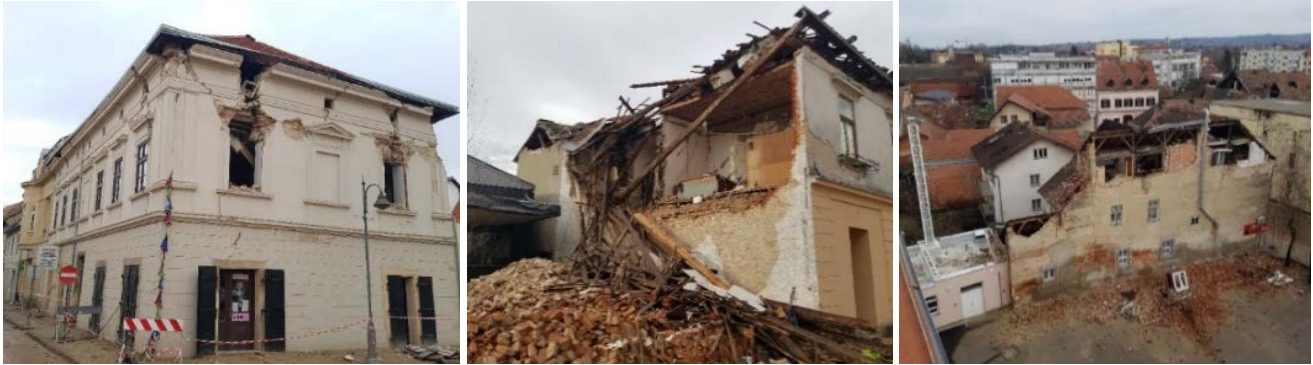
Fig. 5. Petrinja – typical damages [14]
