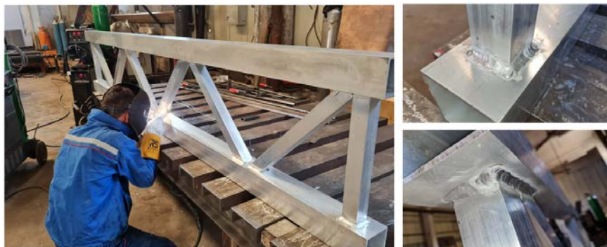
Fig. 4. Welding of aluminum lattice girders
