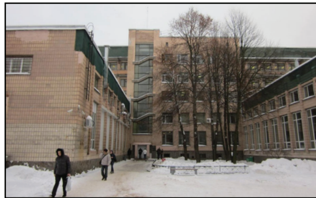
Figure 1: Appearance of the building
