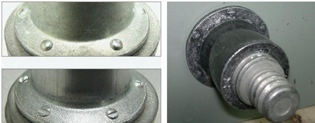
Figure 5: Installation indicators on collar flange before and after installation
