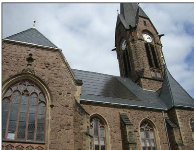
Figure 1 : Herz-Jesu-Kirche in Plauen, photovoltaic systems on the roof of the Lutheran Church in Saxony
