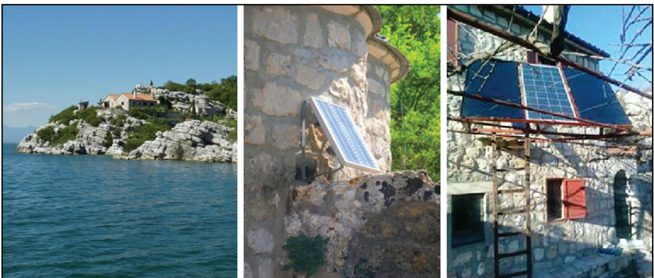
Figure 4: The Starcevo monastery with solar panels mounted on the church walls [16]
