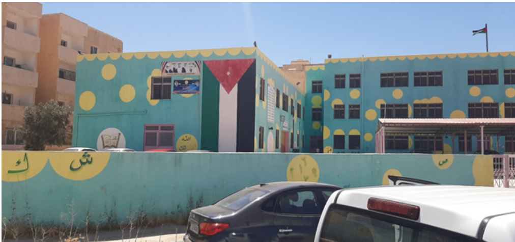
Fig. 1. A north-east exterior view of the school
