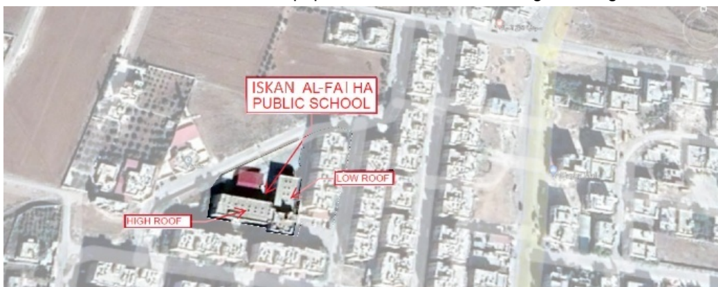
Fig. 2. A satellite image for Iskan Al-Faiha public school (highlighted)-source: [55], located at 31.72° N latitude and 35.78° E longitude, source: [Google Maps], showing the lower roof unit (right) and higher roof one (left) appears in Fig. 1, edited by the 1st author using Adobe Photoshop
