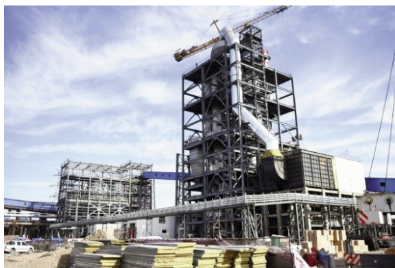
Figure 9. Industrial iron ore magnetizing suspension roasting equipment
