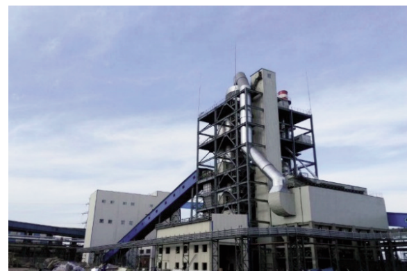
Figure 9. Industrial iron ore magnetizing suspension roasting equipment
