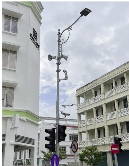
Figure 6. Smart Street Light with CCTV and Horn Speaker in Precinct 15 (Source: Authors)
