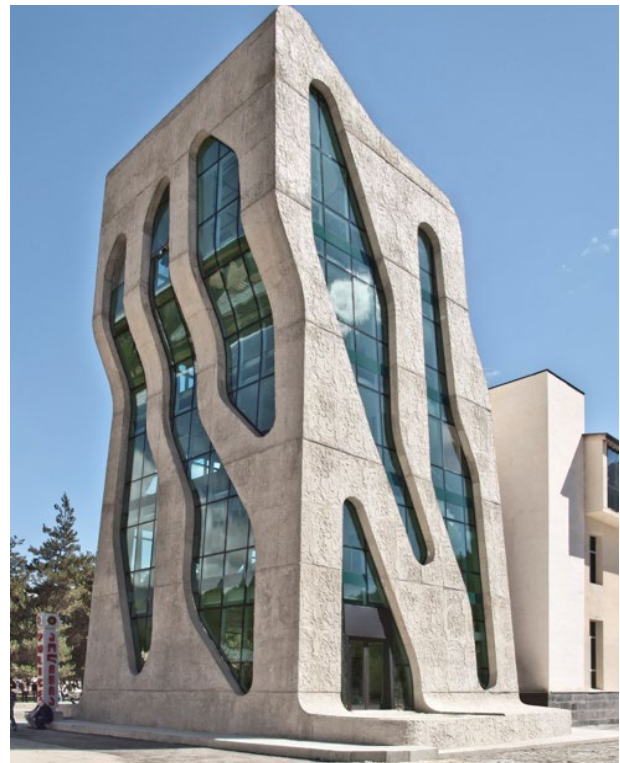
Figure 5: Police Station in Mestia
