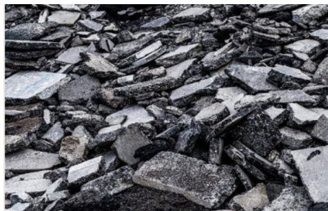
Figure 1 – Milling of existing asphalt pavements
