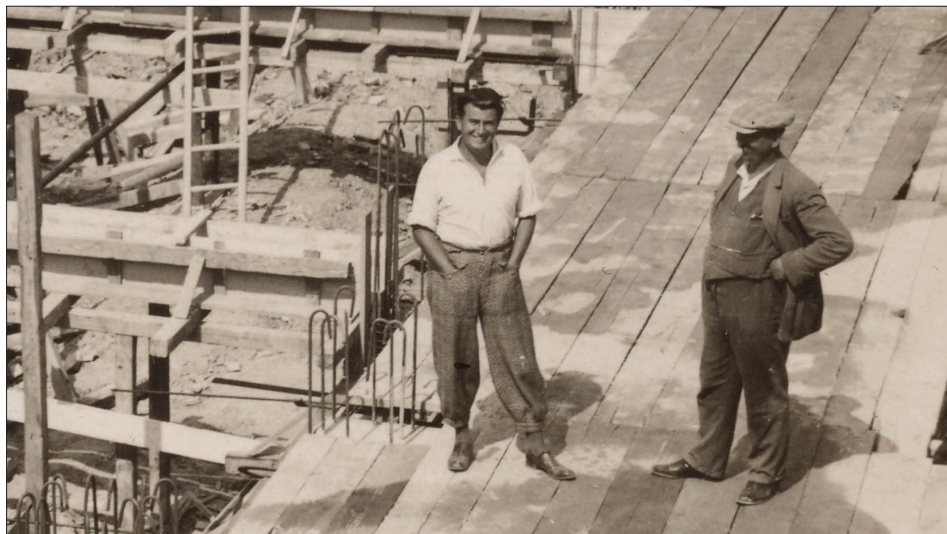
Figure 3. Nikola Dobrović with a worker at the construction site of the Grand Hotel, Lopud near Dubrovnik, 1936. The Museum of Science and Technology, Belgrade.
